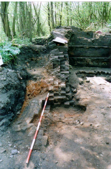
Park Bridge coke ovens
